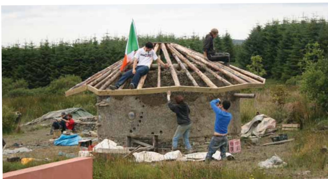
building a cob house at the youth exchange in Co. Clare
